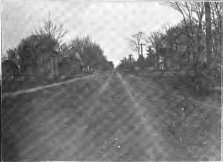
Sea Avenue, Point Pleasant, Ocean Co., after improvement.
